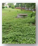
**BEL Machilipatnam Unit:** Three underground rain water storage tanks are constructed to collect rain water from the roofs various buildings inside the factory. The water collected from the roofs of various buildings is connected to underground tanks through PVC pipes. Total capacity of rain water collection in the BEL –MC is 146 KL.
