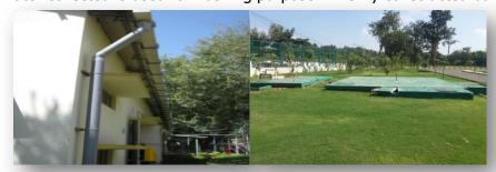
**Rainwater Harvesting Facility:** Large scale RWH reservoir at BEL Bengaluru Unit has a capacity of 170 Million Litres with expected annual yield of around 234 Million Litre. Total enclosed area is around 37,229 Sq. M (10 Acre) with Maximum Water Holding Capacity of 170 ML and Maximum Harvestable Quantity of 235 ML. Project was commissioned in April 2003 at a cost of Rs.57 Lakhs.
