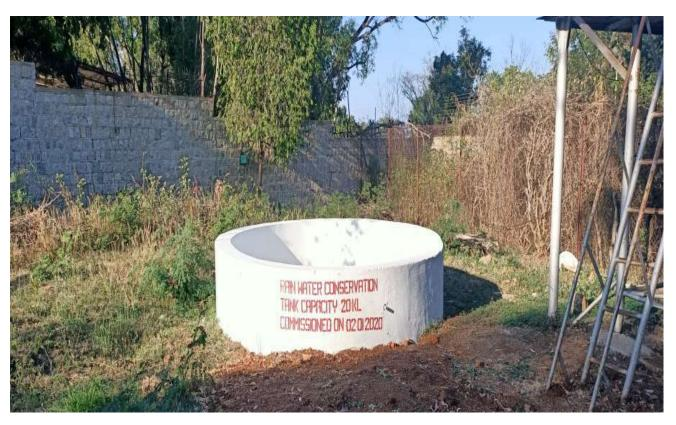
d) Sump Tank has been installed at the test house building for collection of Rain water.
