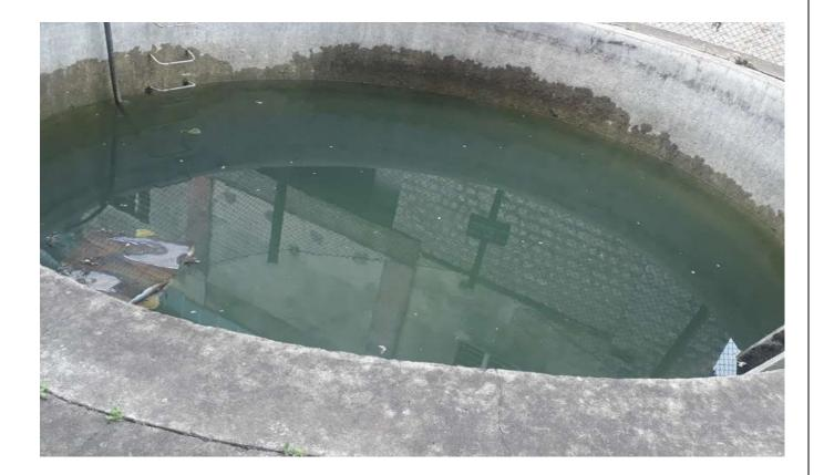
b) At the Old Compressor House in the factory, the Rain water Collection Tank has the capacity of 100000 Litres and the water collected is used for Fire Hydrants in the LPG Yard
