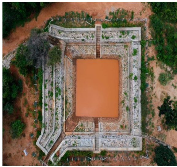
Before and After pics of Water pond
