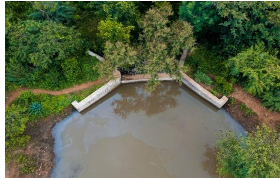
Before and After pics of Check dam
