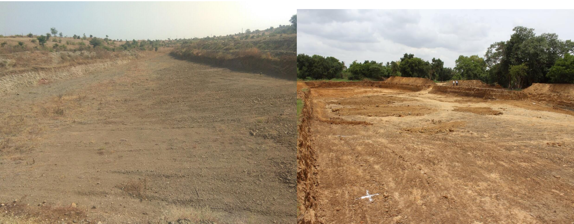
Completed structures before rains
