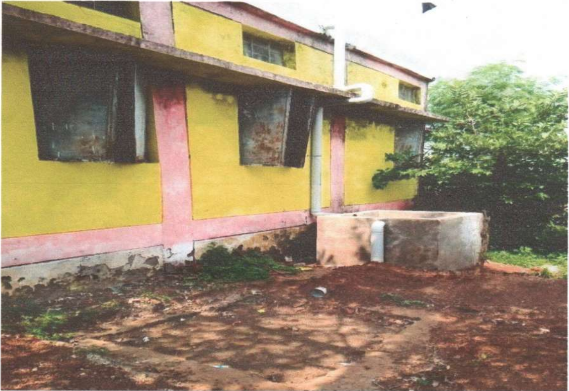
Roof Water Harvesting, Village-Umardeeh,Block- Mohgaon, Distt.-Mandla.
