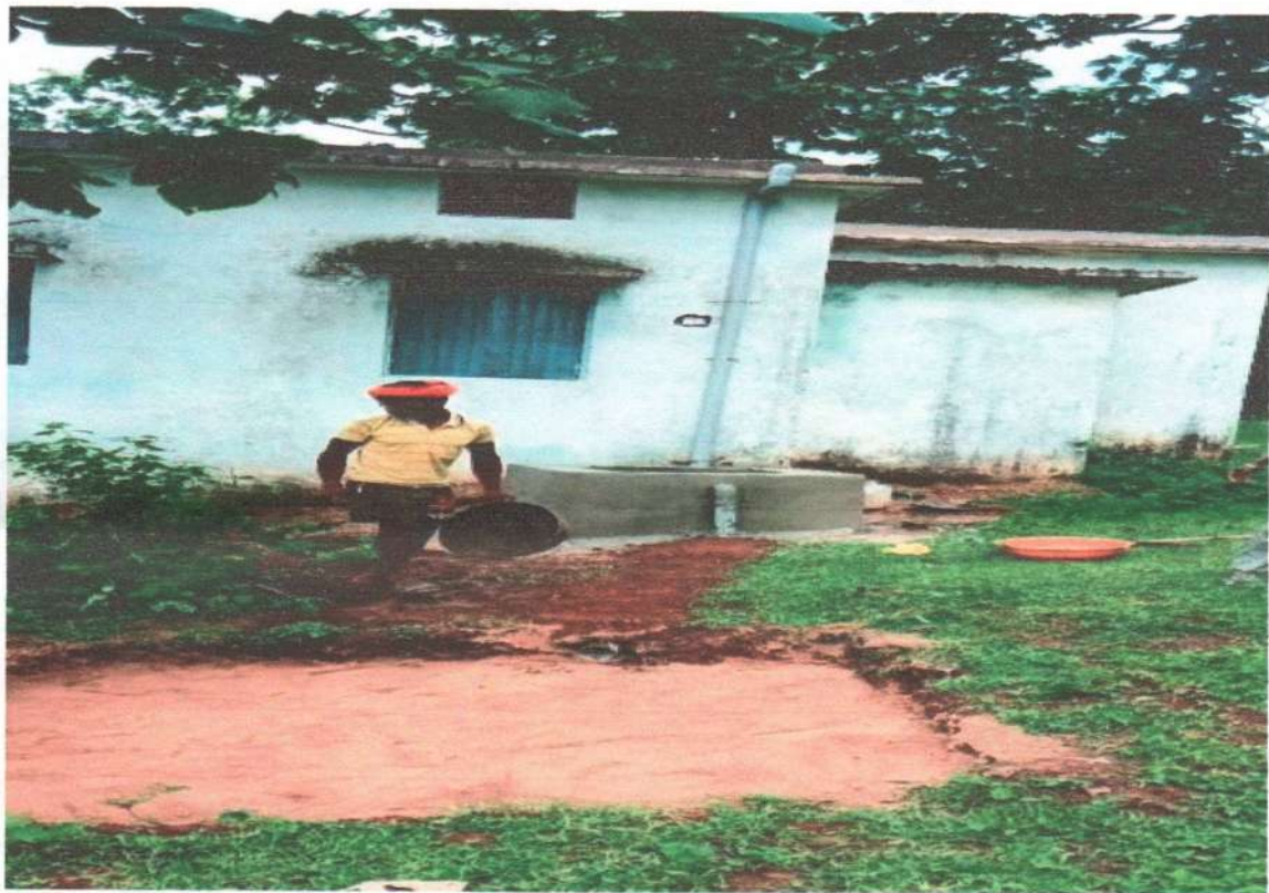
Roof Water Harvesting, Village-Chubhaaval, Block- Mohgaon, Distt.-Mandla.
