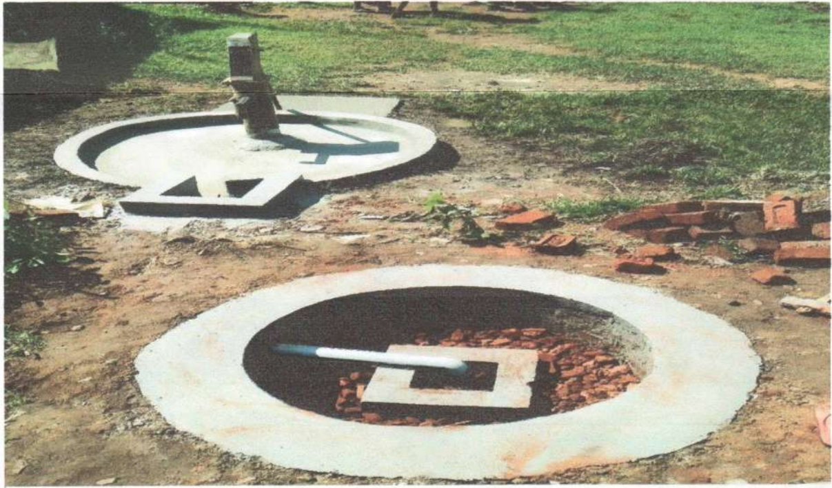
Soak Pit, Gram- Malvathar, Block- Mohgaon, Distt.-Mandla
