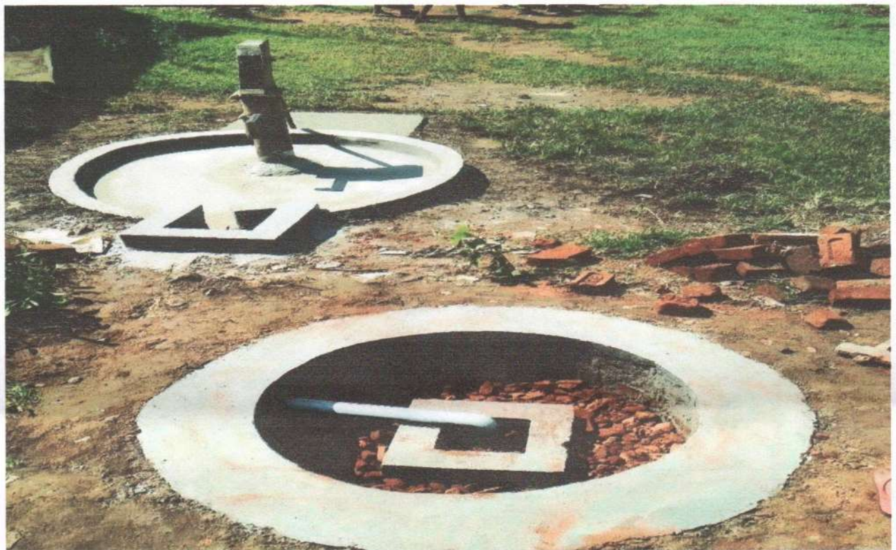
Soak Pit, Village-Malvathar, Block-Mohgaon, Distt.-Mandla
