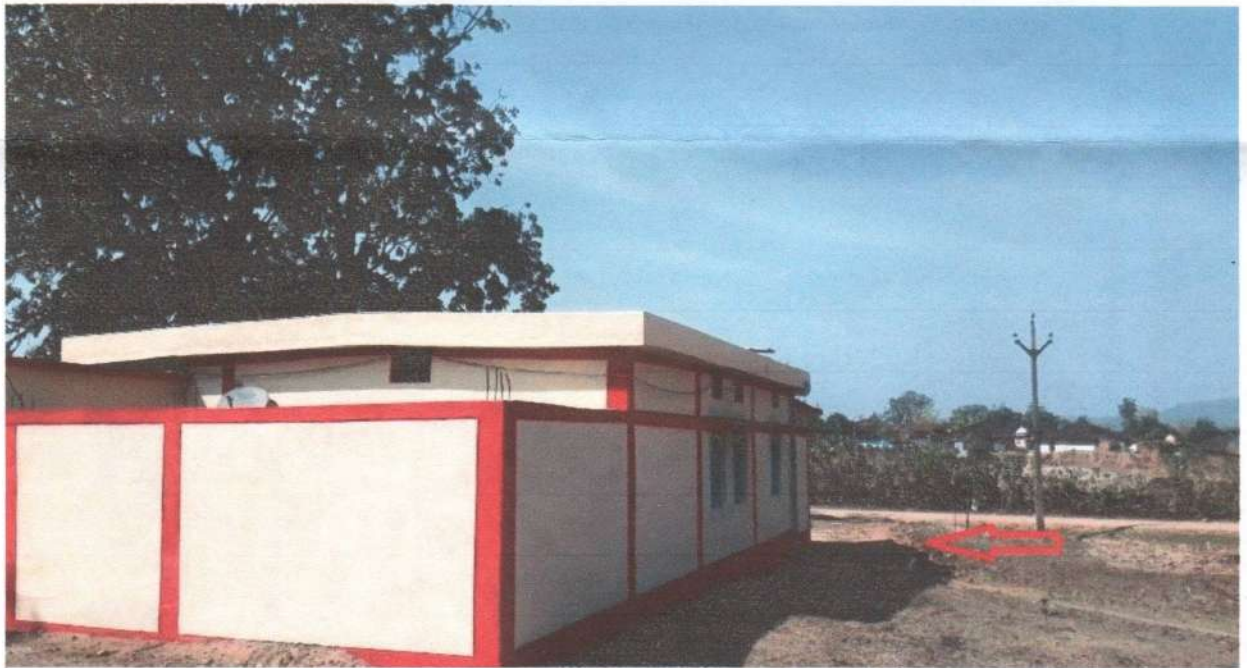
Roof Water Harvesting, Village-Pandiwara,Block- Nainpur, Distt.-Mandla.
