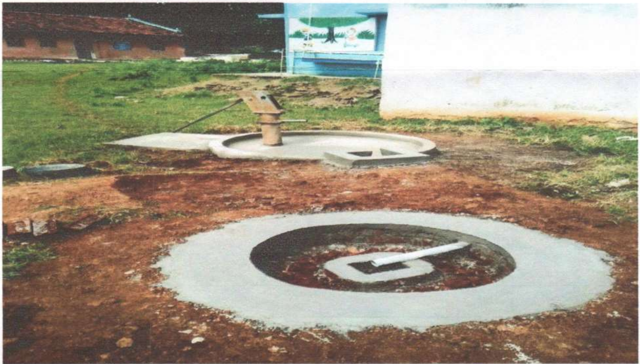
Soak Pit, Village-Malvathar, Block-Mohgaon, Distt.-Mandla
