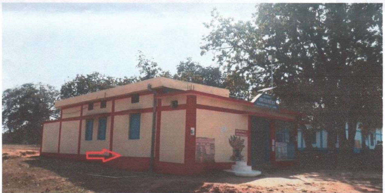
Roof Water Harvesting, Village-Pandiwara,Block- Nainpur, Distt.-Mandla.
