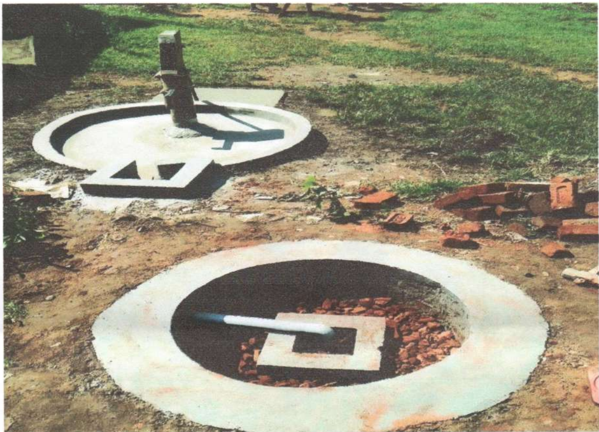
Soak Pit, Village-Malvathar, Block-Mohgaon, Distt.-Mandla
