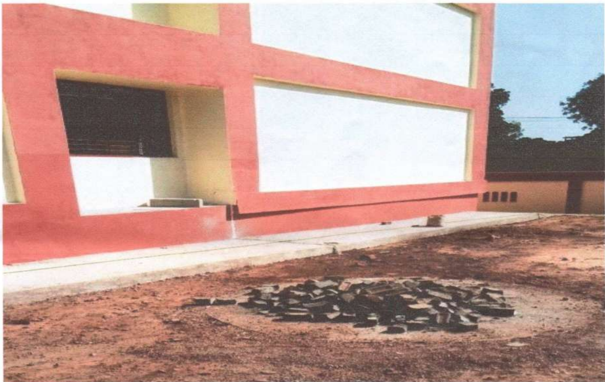
Roof Water Harvesting, Computer Skill Village Katra, Block- Mandla, Distt.-Mandla.
