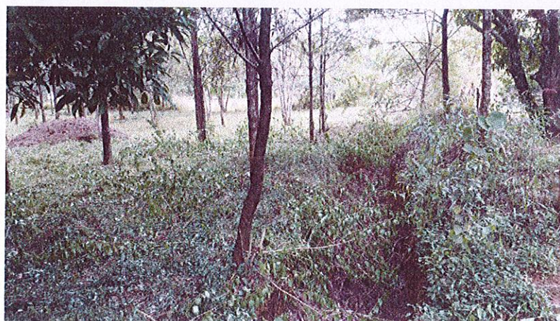
Trenches for Rainwater harvesting
