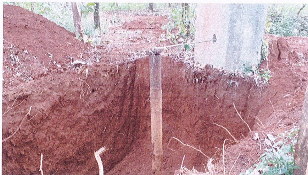
Work in progress for Rainwater harvesting to recharges Bore wells
