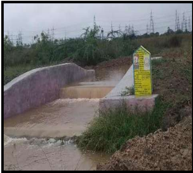
f. Check Dam after
