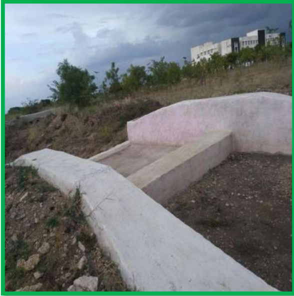
e. Check Dam before
