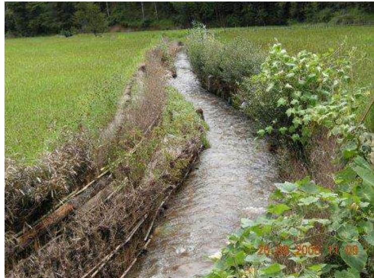
Traditional irrigation and indigenous management to check bank erosion using locally available materials
