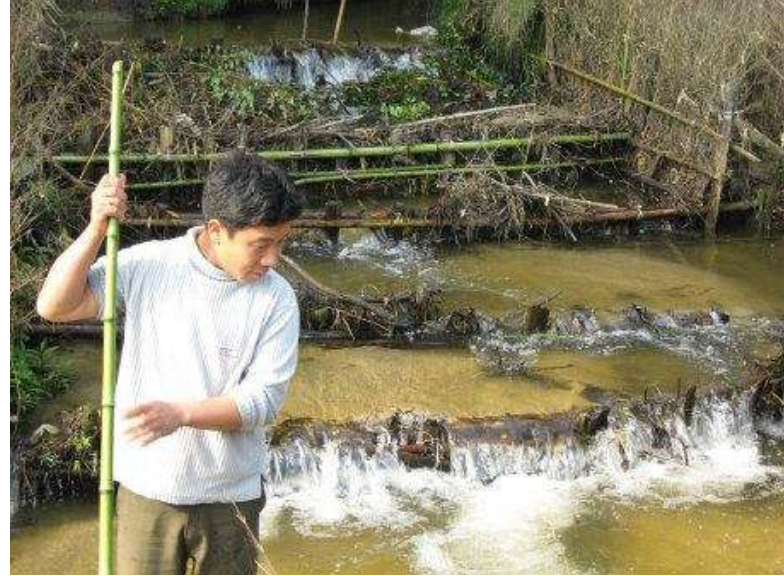
Traditional check dam of Apatani is the unique system of traditional irrigation known as Bogo.
