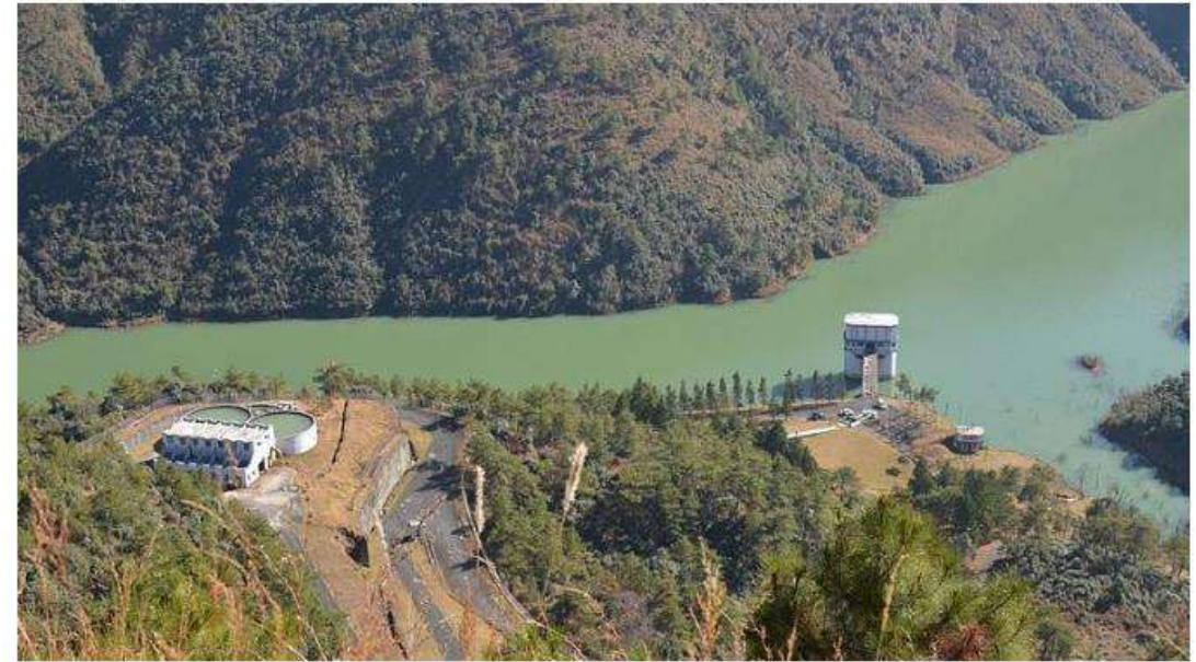
The reservoir at Mawphlang. Pic: Flickr/CC BY 2.0
