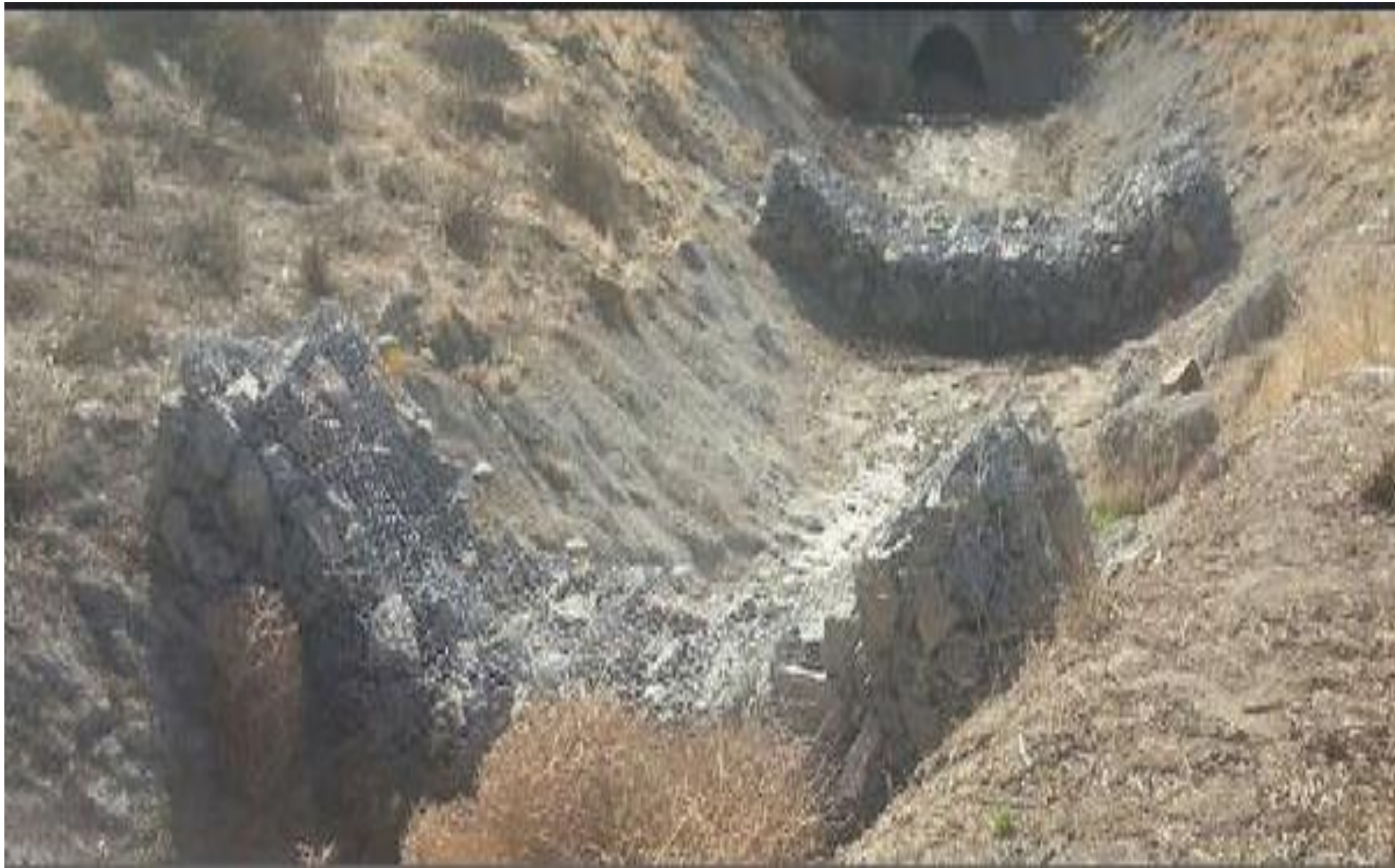
Gabion Check Dam
