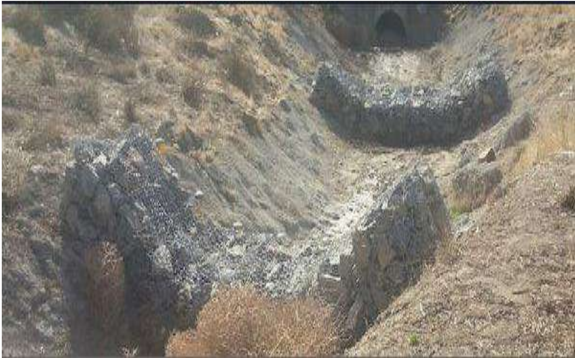
Gabion Check Dam
