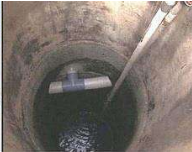
Use of Abandoned dugwells
