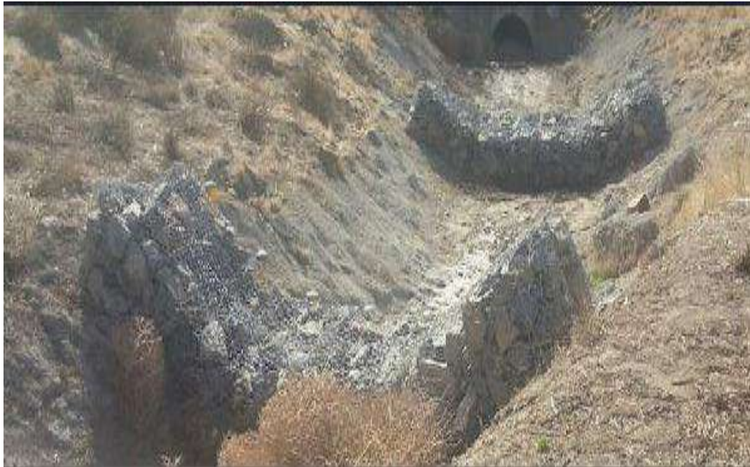
Gabion Check Dam
