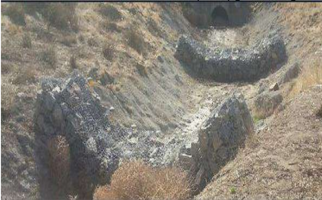
Gabion Check Dam
