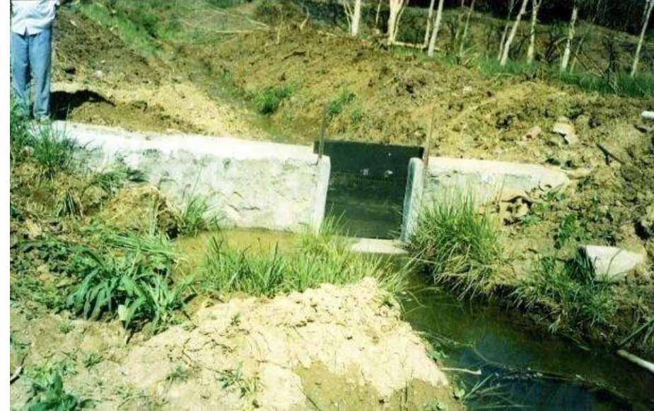
Check Structure in canal escape
