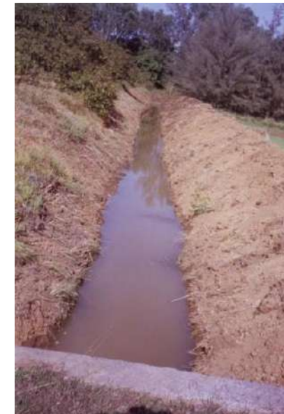
Water storage behind the check dam
