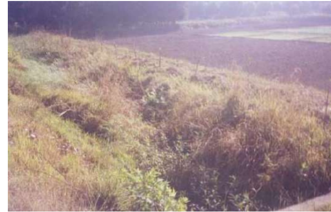
Chocked canal escape
