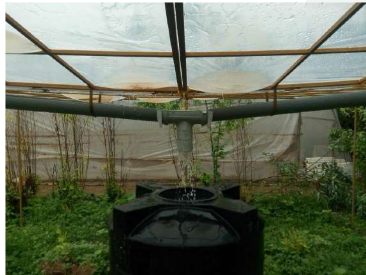
Portable Water Harvesting Structure
