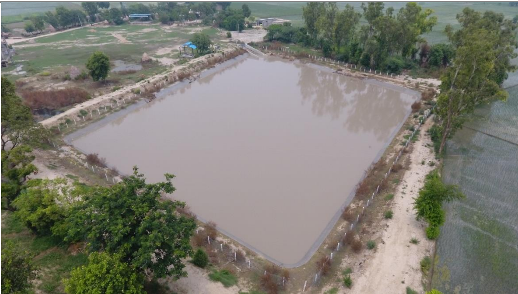
Rainwater Harvesting Site at Punjab-Phumanwal
