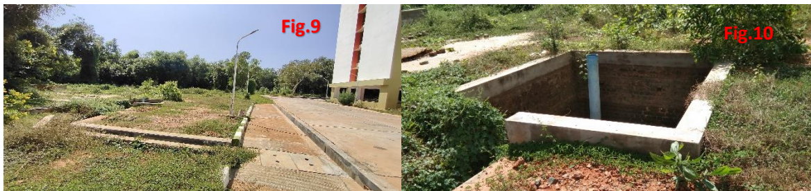
Fig.9 &10 Roof Top harvesting structures
